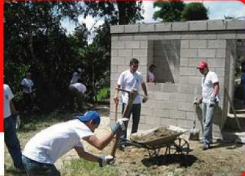
Volunteers help in construction of school.
